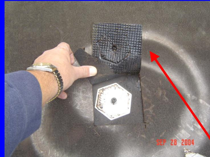
Here the contractor did not install a cover board insulation, adhere the base sheet to the insulation and did not even melt the torch applied modified bitumen membrane. This roof flaps in the wind.
