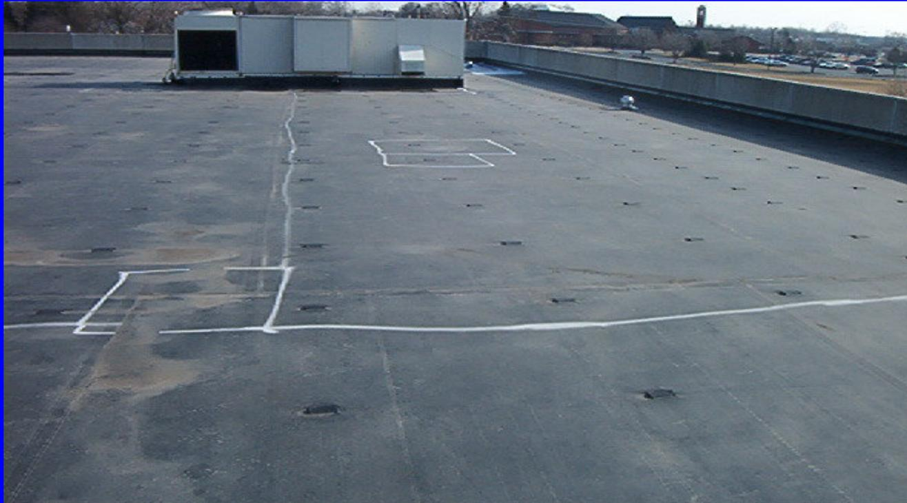
Fasteners clip plates were installed too tight resulting in tears around fasteners.
